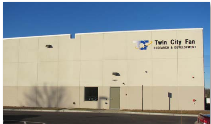
Minneapolis, MN Research and Development Lab
