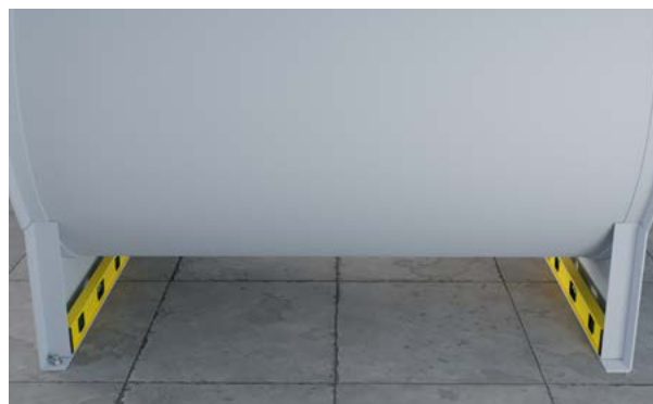
Carefully level the fan on the foundation
