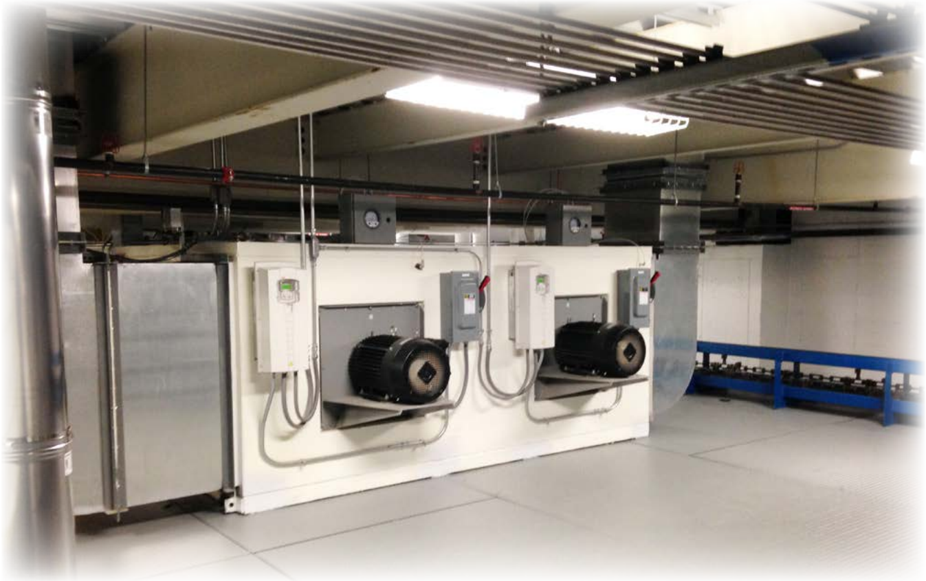
Recirculation Fans in Paint Finishing System
