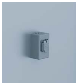
NEMA 1 Disconnect Switch
