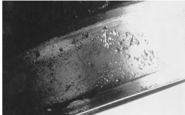
Figure 7. Spalls & Wear Patterns in the Race
