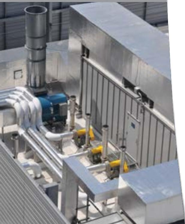
room noise criteria inside the facility. Additionally, exhaust fans either located outside of the building or ducted to the outside must meet community noise levels. The supply fans used in the generator room also required silencers to prevent transmitting generator noise to the outside.
