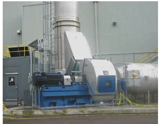
Insulated fan used for an RTO application
